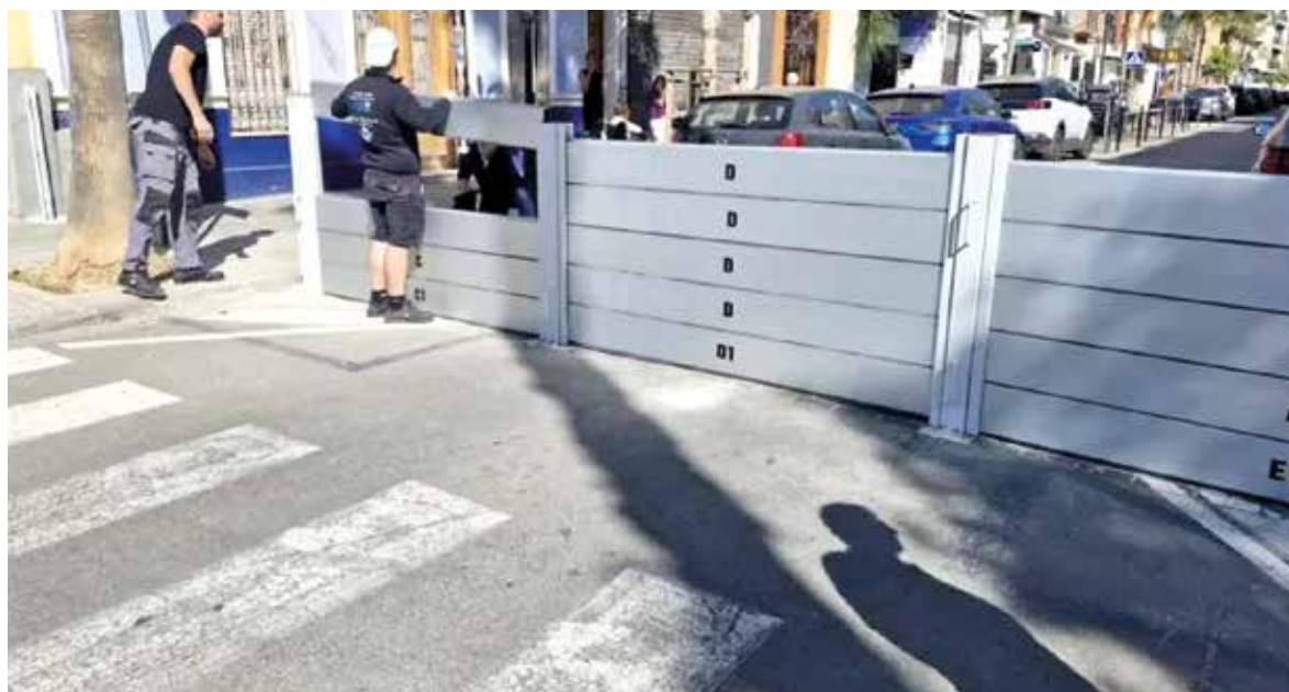
Noves comportes a Aldaia
